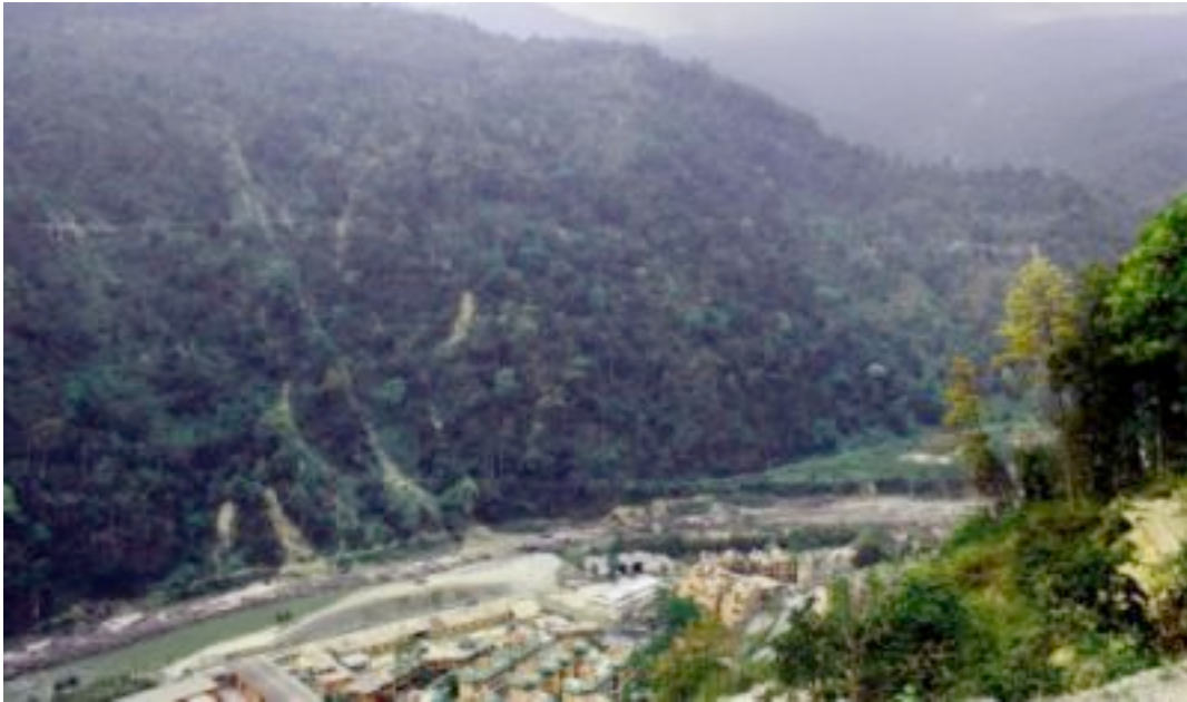
The power house of the Teesta Phase 5 project.
