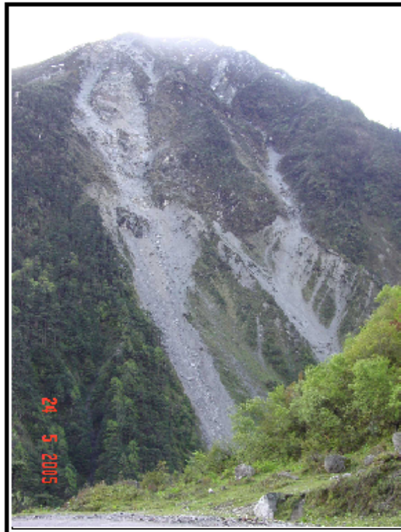
Plate 2.21 Landslide along the left bank of Teesta in Lachen axis
