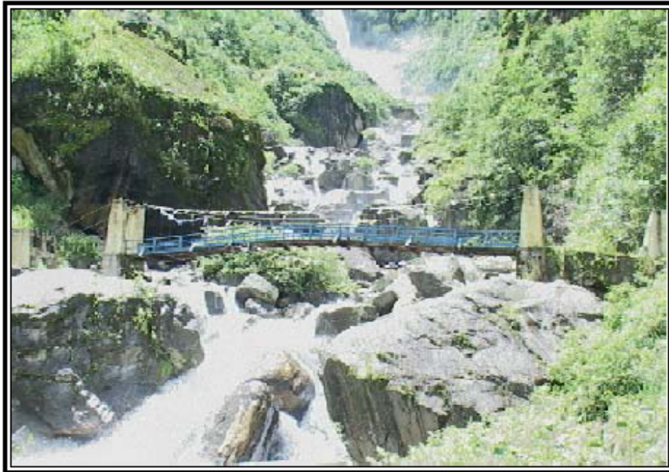
Plate 2.9 Water dashing at high velocity at Ri Chhu landslide site
