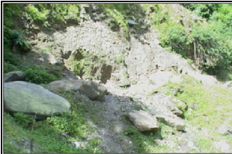
Plate 2.12 Collapse of old terrace and landslide cones at Tong
