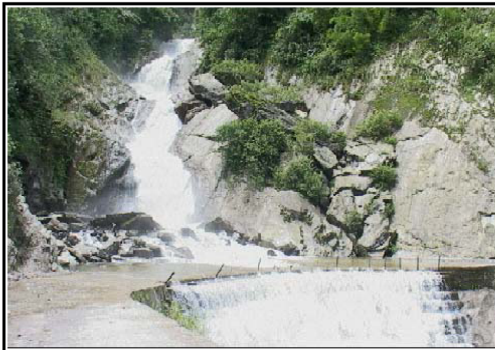
Plate 2.8 Myang Khola Landslide
