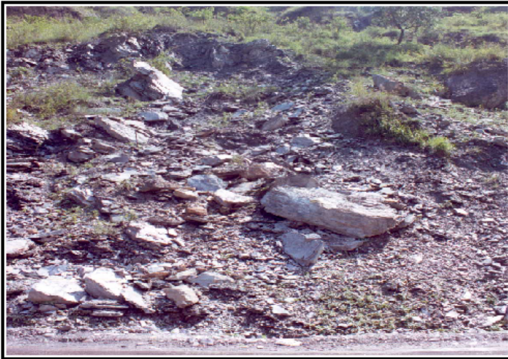
Plate 2.15 Rangpo landslide showing Rock fall and debris flow
