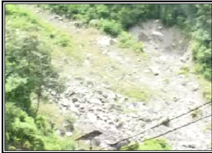
Plate 2.7 Lanta Khola Landslide
