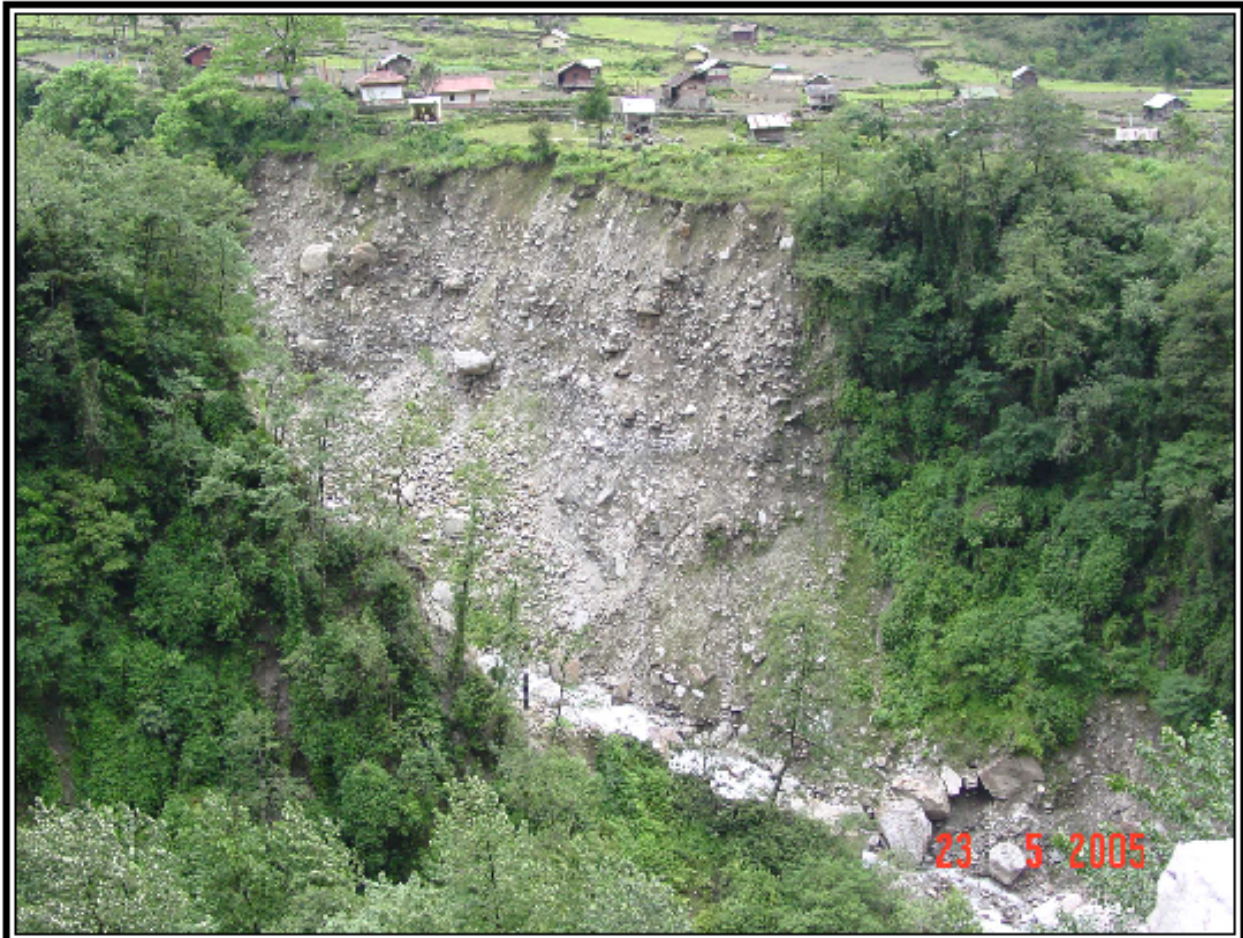
Plate 1.10 Collapse of Terrace on the left bank of Lachung and Creeping of settlement on it
