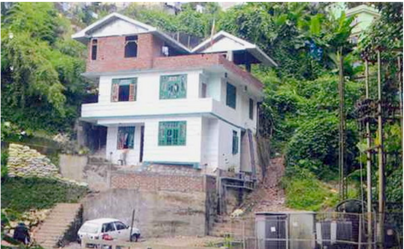
Much repaired - SDF prez Chumbey Rai's house
