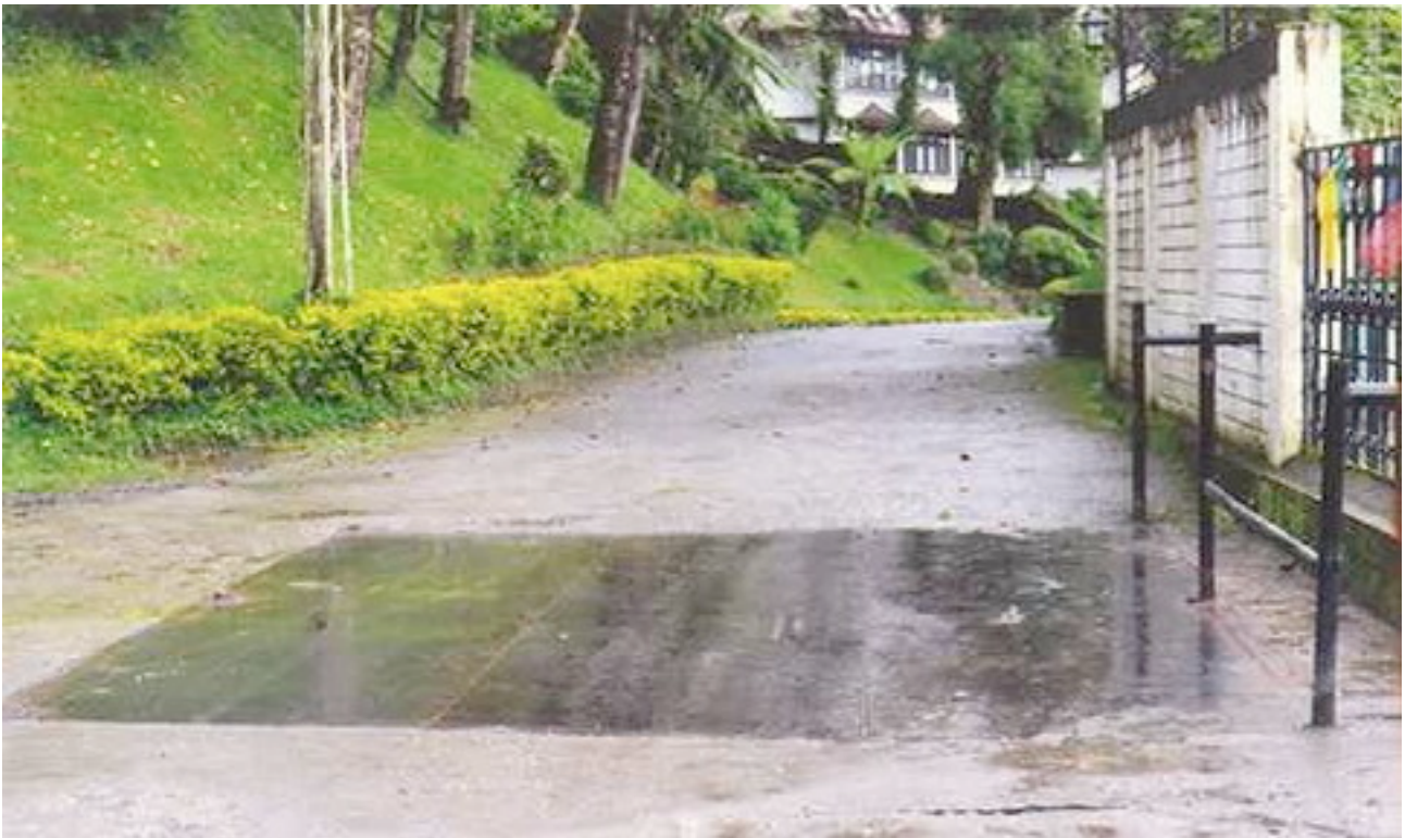
Wrong approach - The steel 'bridge' on Norkhil Jhora
