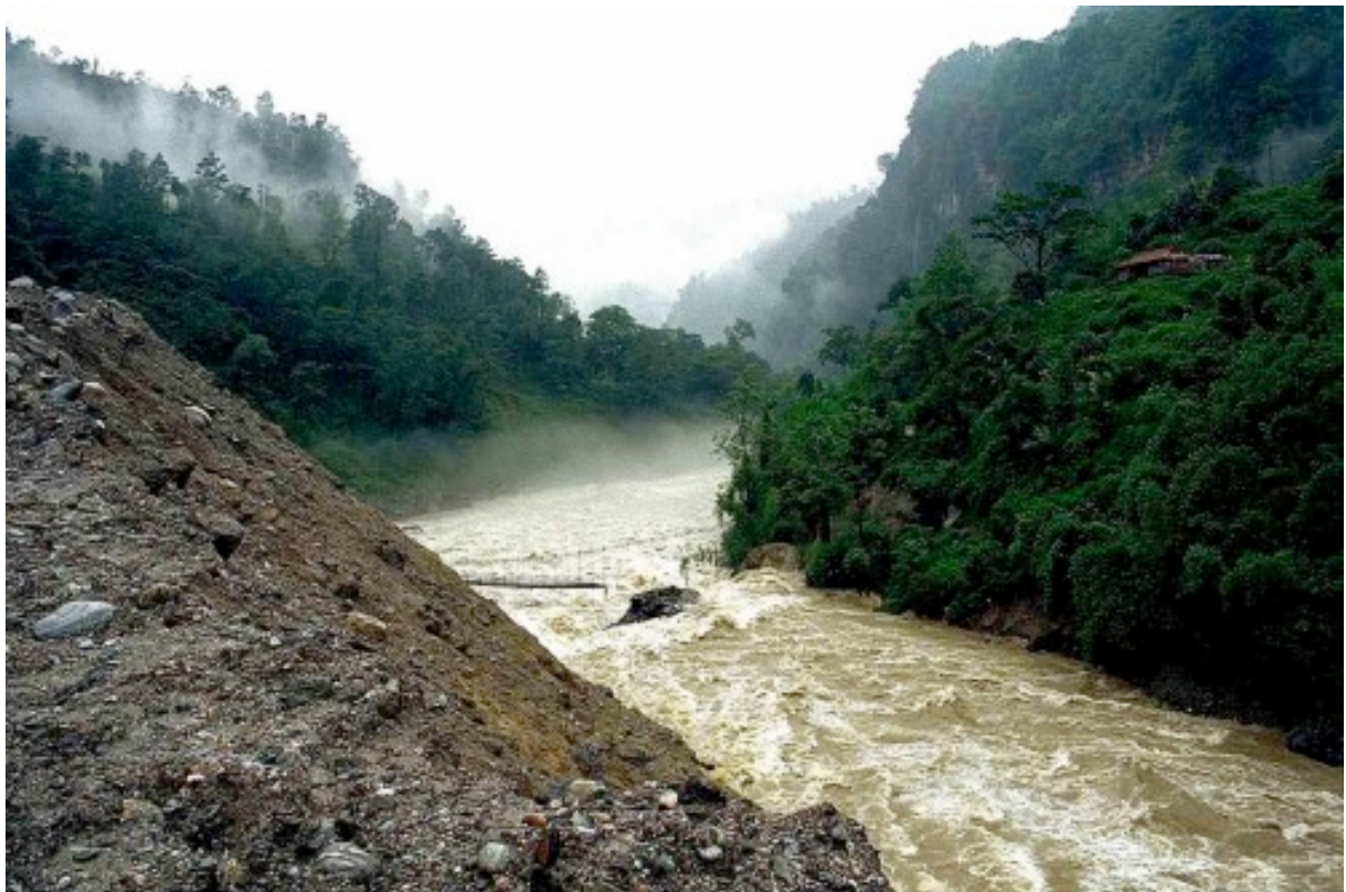
Muck and debris from the Teesta V project being dumped in the river. (Photo by Manju Menon)
