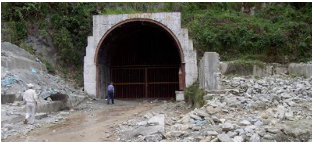
One of the tunnels at the Teesta River
