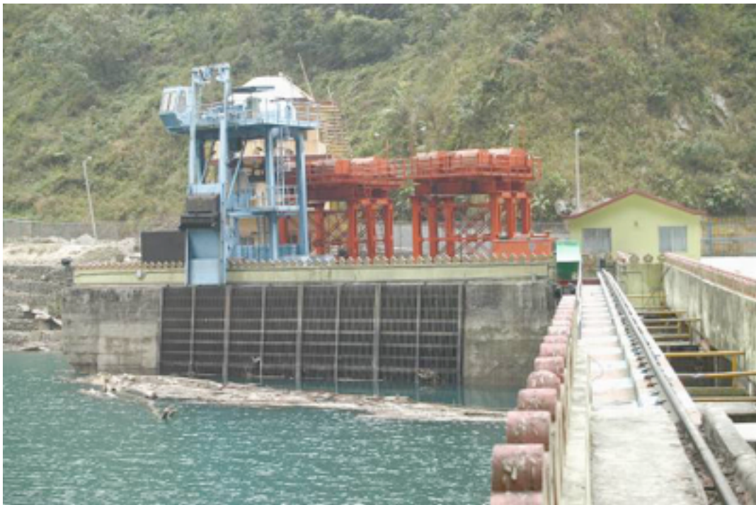
The 60 MW Rangit Power House Source: Government of Sikkim
